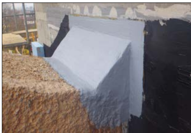
Component connection/surface seal
