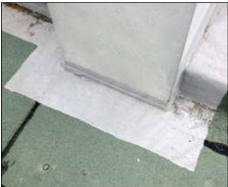
All pictures on this page: sealing of threshold connections and material transitions
