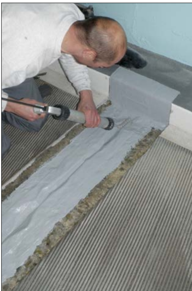
Movement joint/dilatation joint
