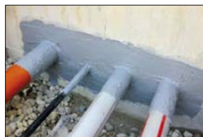
Component connection/surface seal
