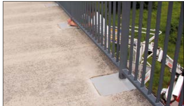
A11 Motorway/Germany: Bridge cap and walk way renovation
