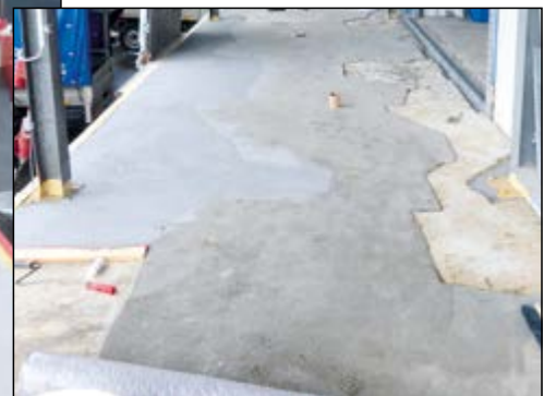
Forwarder warehouse, Kassel/ Germany: Renovation of a loading ramp
