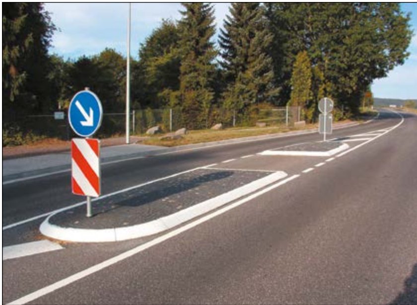
K 106 by-road, Neuwied-Niederbieber/Germany: Kerb of a traffic island stuck to the asphalt with SILIKAL® R 17 mortar
