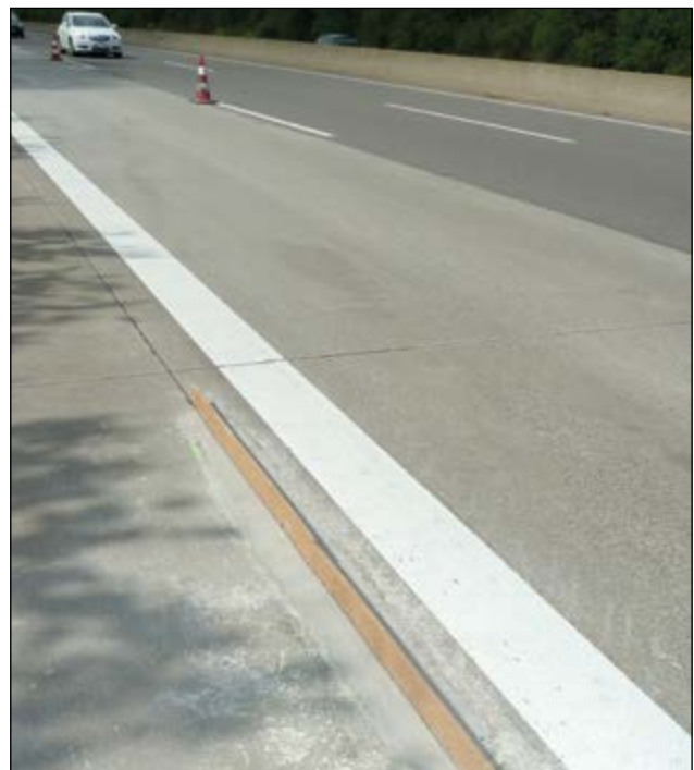
A4 Motorway near Düren/Weisweiler/Germany: Concrete slab edge repair
