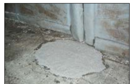
Figure on top: Deutsche See GmbH & Co. KG, Bremerhaven/Germany: Repair of floor areas in cold store house with SILIKAL® R 17 mortar with no disruption to operation (-25 °C)
