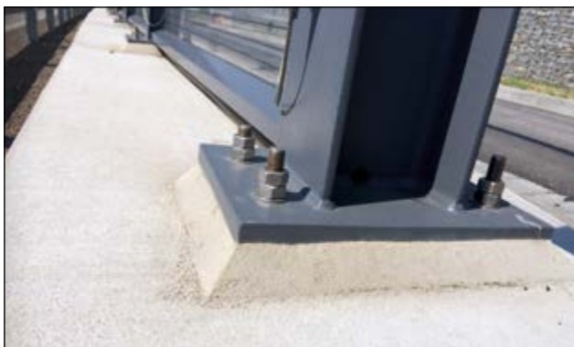
B42 Interstate Road/Germany: Underlayment of steel construction
