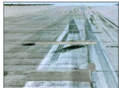
Leipzig/Halle Airport/Germany: Repairing concrete, runways and taxiways
