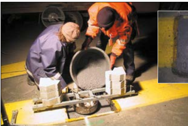
Nordrhein-Westfalen Airport/Germany: Replacing and installing embedded runway lights without air-traffic interruption
