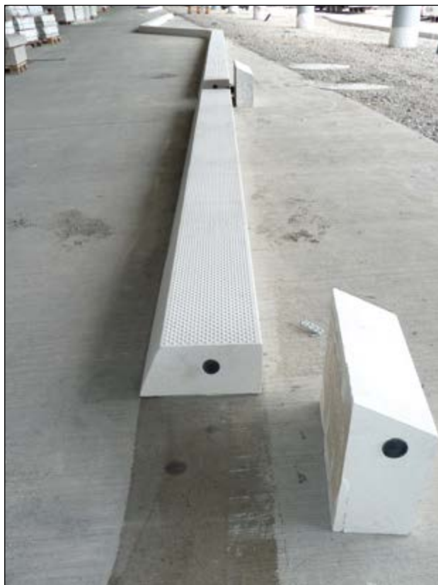
Car park airport, Stuttgart/Germany: Kerb stone stuck to concrete with SILIKAL® R 17-thix mortar
