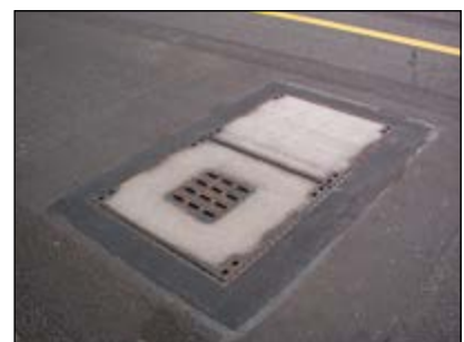
Nordrhein-Westfalen Airport/ Germany: Sealing cable ducts with asphalt- coloured SILIKAL® R 17 mortar
