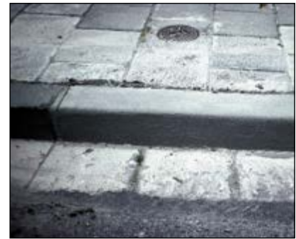
Repairing the kerbs with SILIKAL® R 17 mortar
