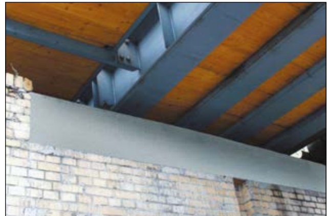
Metropolitan viaduct, Berlin/Germany, Sterndamm: repairing bridge bearings
