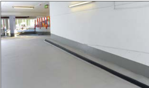
Car park "Altlohrtor", Koblenz/Germany: Renovation of ramps
