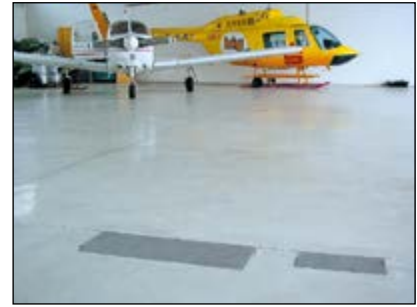
Mannheim Airport/Germany: Repairing hangar floors
