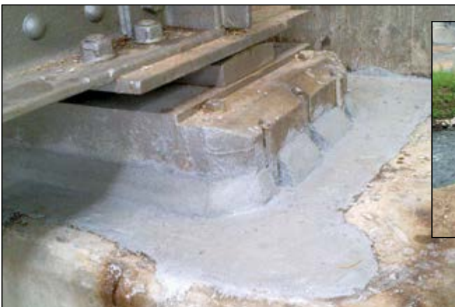
A6 Motorway Bridge, Massholdertal/Germany: New bridge bearings
