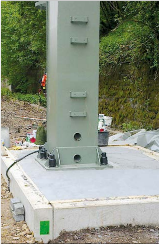
Railway track Düsseldorf-Wuppertal/Germany: Installation of steel columns
