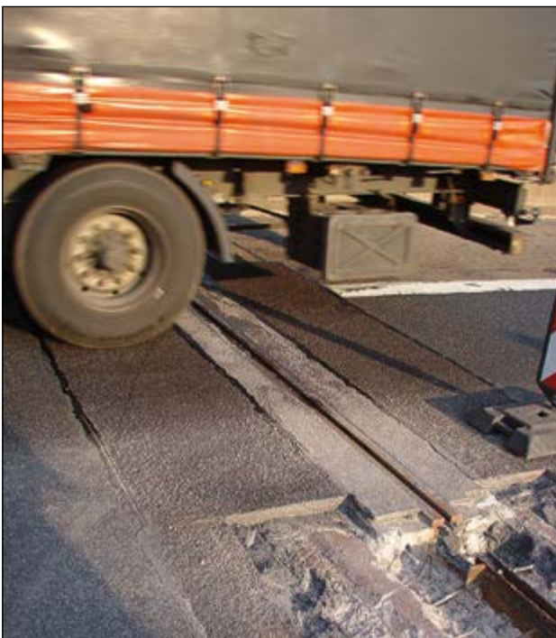
A45 Motorway near Solms/Germany: Repair and implantation of joint profiles
