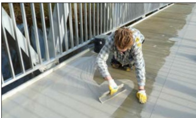
Wied-Bridge, Waldbreitbach/Germany: Surface coating of an aluminium pedestrian bridge
