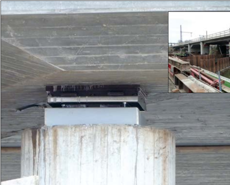
New railway bridge construction in Hannover-Ohedamm/Germany: Bridge bearings
