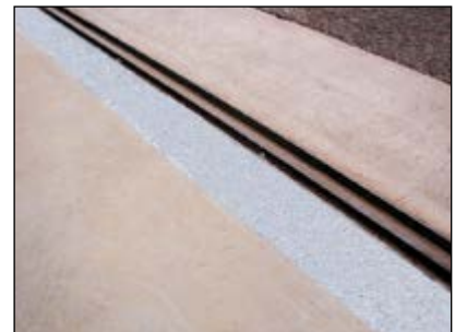
Mannheim Airport/Germany: Laying foundations of sliding door rails
