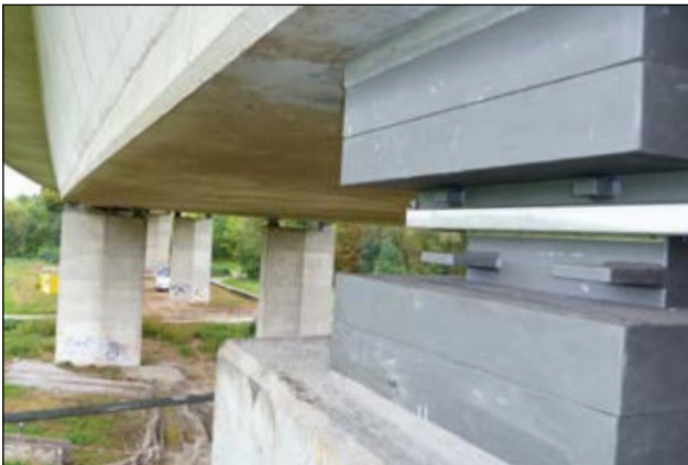
A6 Motorway Bridge, Massholdertal/Germany: New bridge bearings
