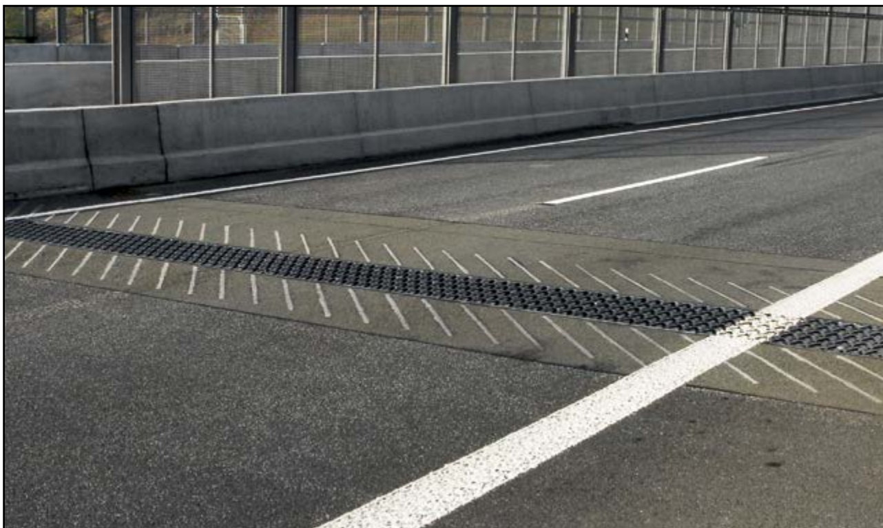
A38 Motorway near Breitenworbis/Germany: Joint rip profile installation
