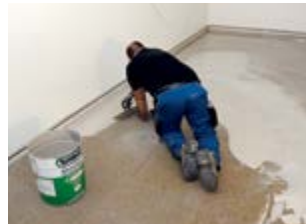
Application of main coat
